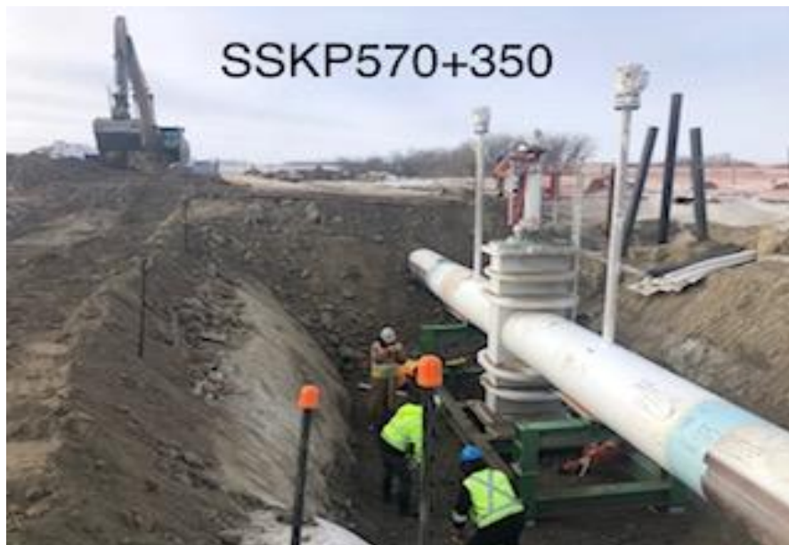
MLBV15 Compaction lift process- worker remove clay/ rocks from the excavation
