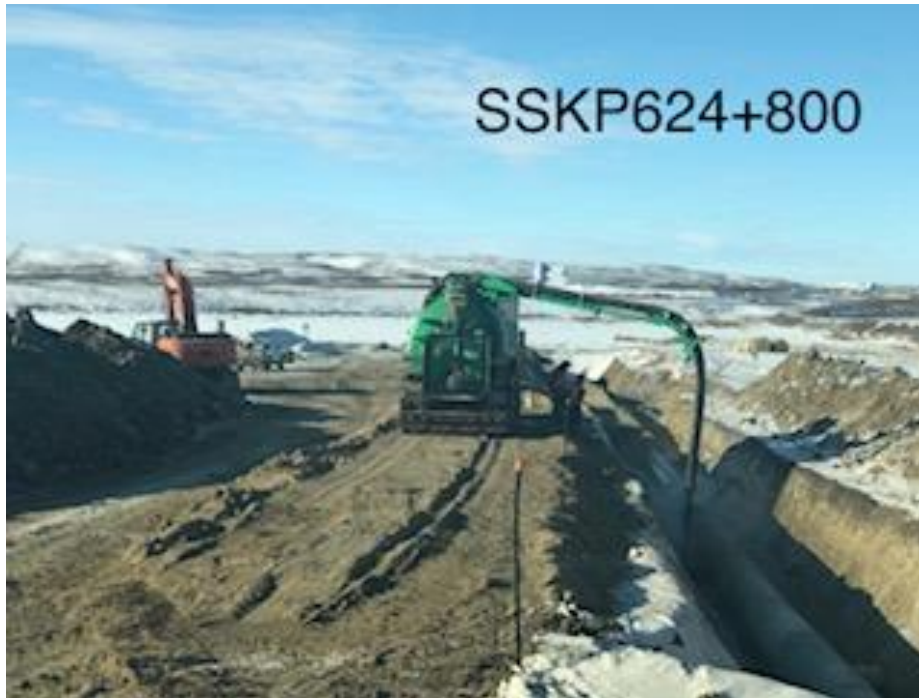
Hydro vac clearing ice from around the pipeline before shading in
