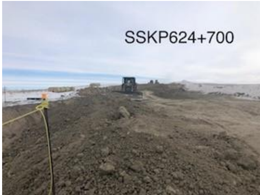
Shading in and backfill ongoing at east side of Chapleau Lake
