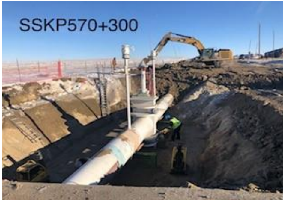
MLBV15 compaction in progress utilizing compaction plates
