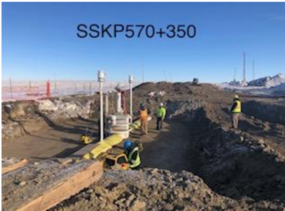
MLBV15 compaction in progress
